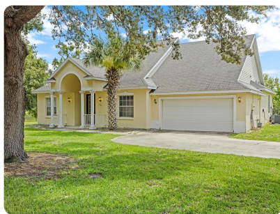
404 Bridgewater Boulevard, Davenport, FL 33896 Compass
