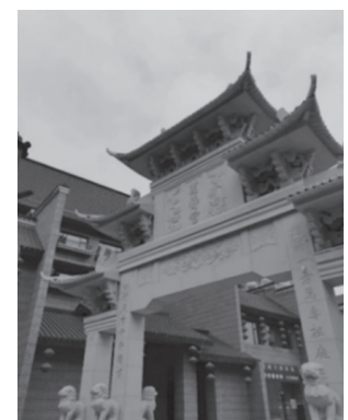
Fig.9 Stone archway at the exit of the street
