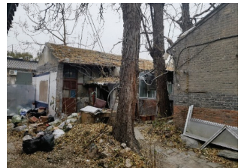
Fig.7 Current situation inside Fengcheng Guild Hall
