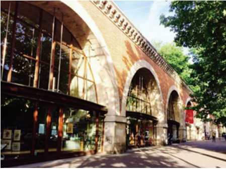
Fig.1 Stores under the Bastille viaduct
