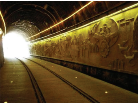
Fig.4 Xiamen Railway Cultural Park Hongshan Tunnel
