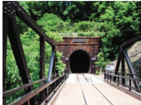
Fig.5 Great Sun Shadow Railway Tunnel in Japan
