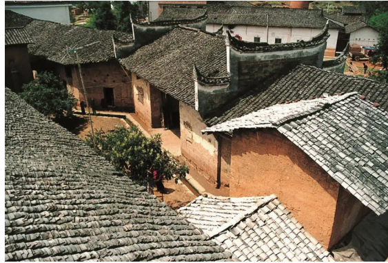
Fig.2 Rammed earth buildings in Shen's Grand Courtyard
