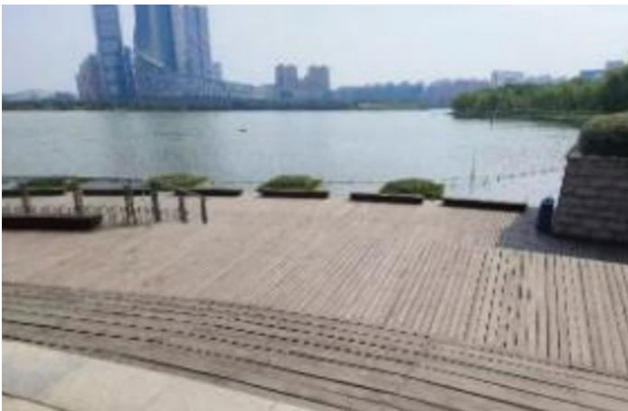
Fig.5 Hydrophilic platform walkway
