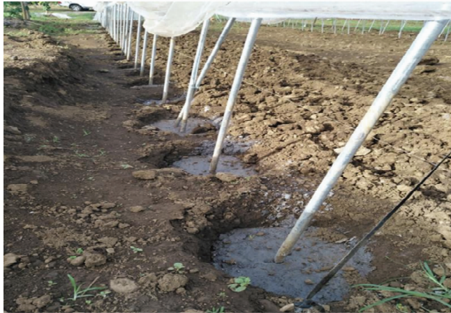
Fig. 2 Reinforcement of greenhouse stand columns
